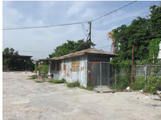
40 Foot Container (security office)
