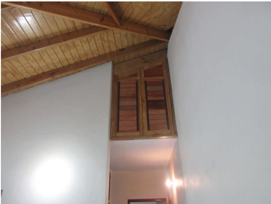
Rear bedroom: View of attic storage door
